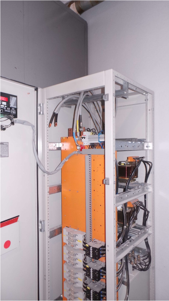
Power factor compensation 100 kVar
